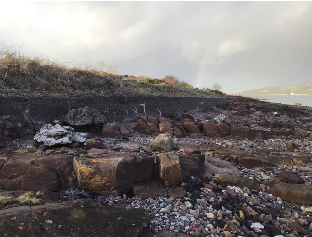
Photograph 11: Seawall, bedrock (sandstone) and cobble upper shore south of the slipway
