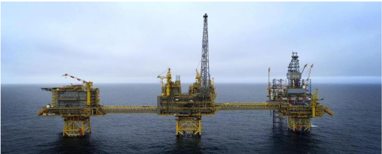
Figure 14 The Culzean platform complex
