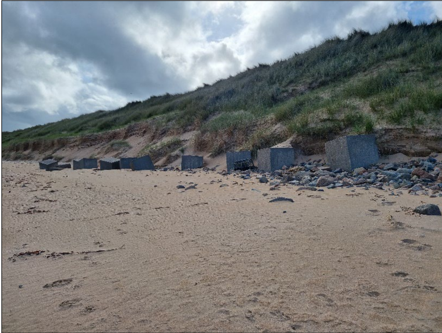
Photo 3: Anti-tank Blocks (TI_034).
