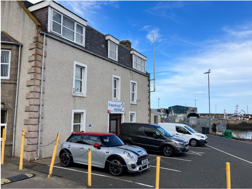
PLATE B. 33: THE HARBOUR WORKS OFFICE AT FRASERBURGH HARBOUR
