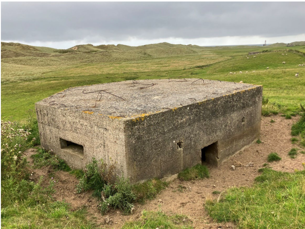
PLATE B. 2: PILL BOX SM11317. VIEW SOUTH-EAST TOWARDS BEACH AND RATTRAY HEAD
