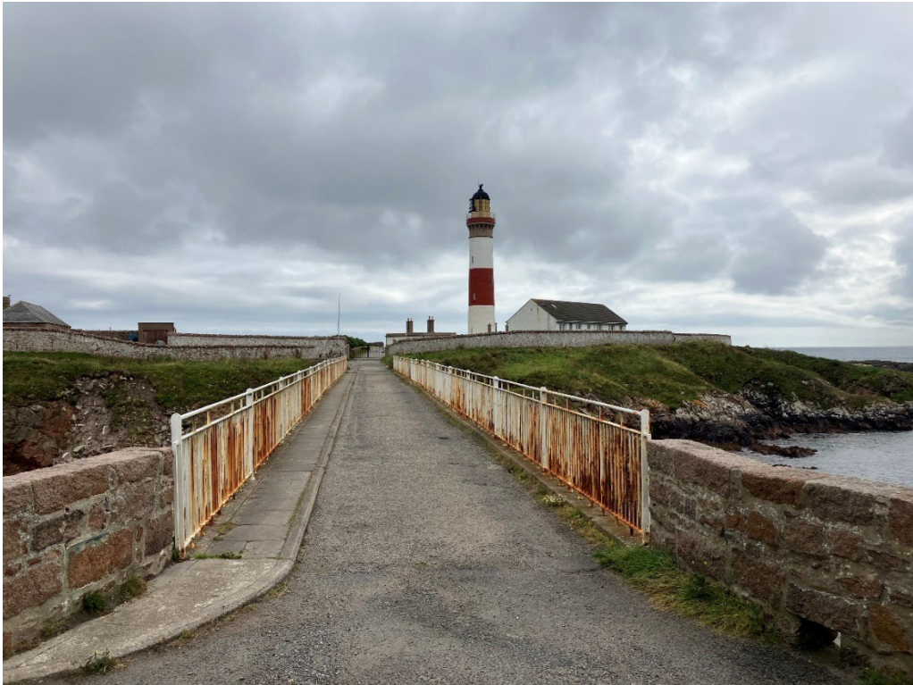
PLATE B. 27: BUCHAN NESS LIGHTHOUSE AND ASSOCIATED BUILDINGS
