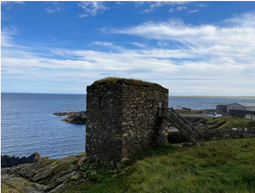
PLATE B. 11: THE WINE TOWER AT FRASERBURGH VIEW SOUTH-EAST TOWARDS COASTLINE AND OFFSHORE ARRAY AREA
