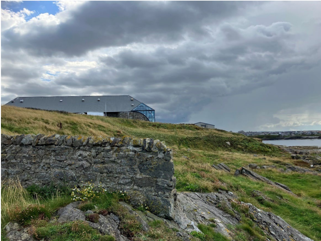
PLATE B. 19: VIEW OVER FRASERBURGH BROADSEA CONSERVATION AREA AND COASTLINE FROM KINNAIRD HEAD LIGHTHOUSE
