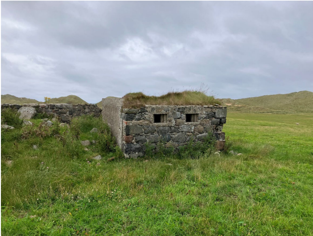
PLATE B. 3: PILL BOX SM11319 SHOWING CONSTRUCTION INTO EXISTING FARMSTEAD BUILDINGS
