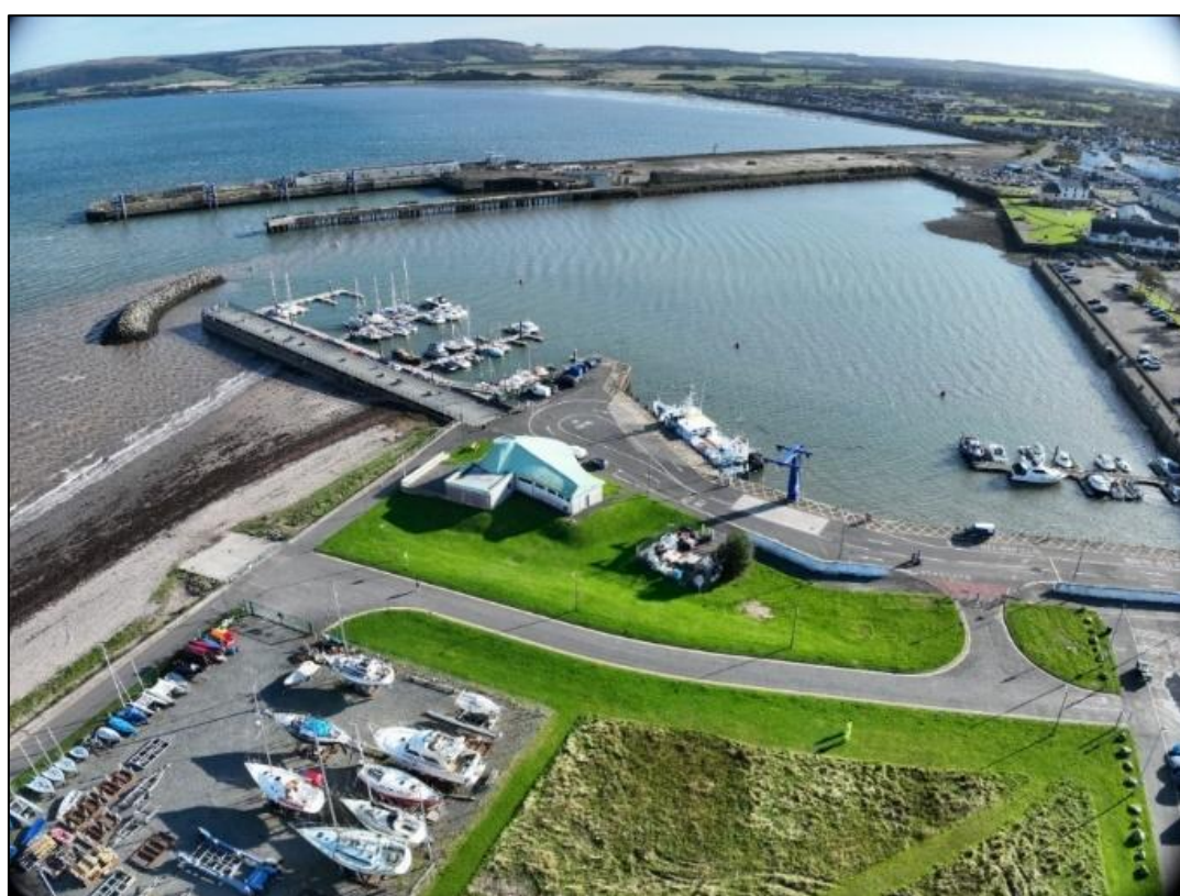
Photograph 10: Existing Modified Harbour Area
