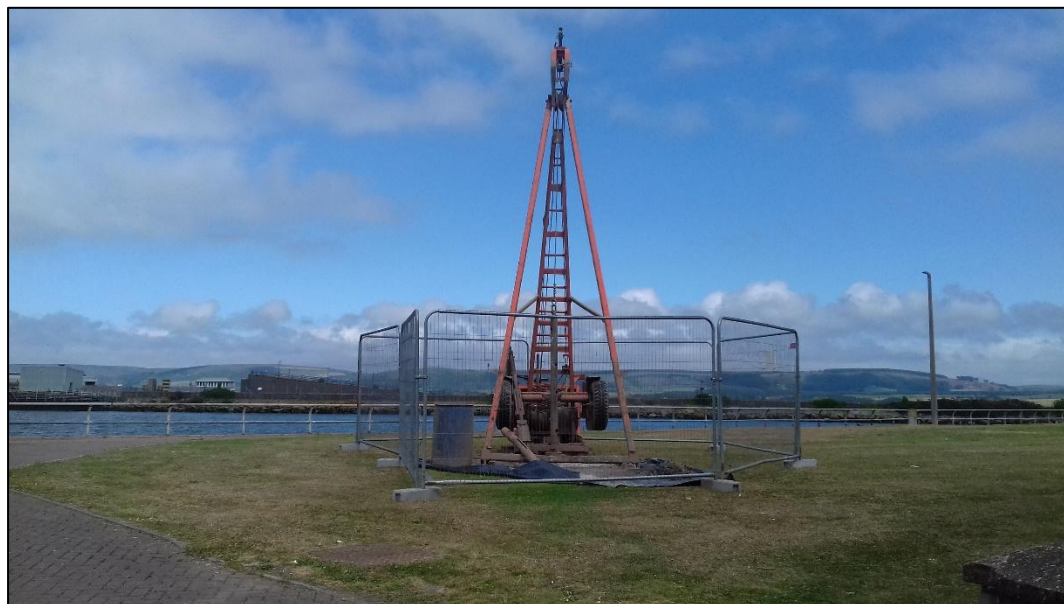
Photograph 13: Apparatus used to establish ground conditions
