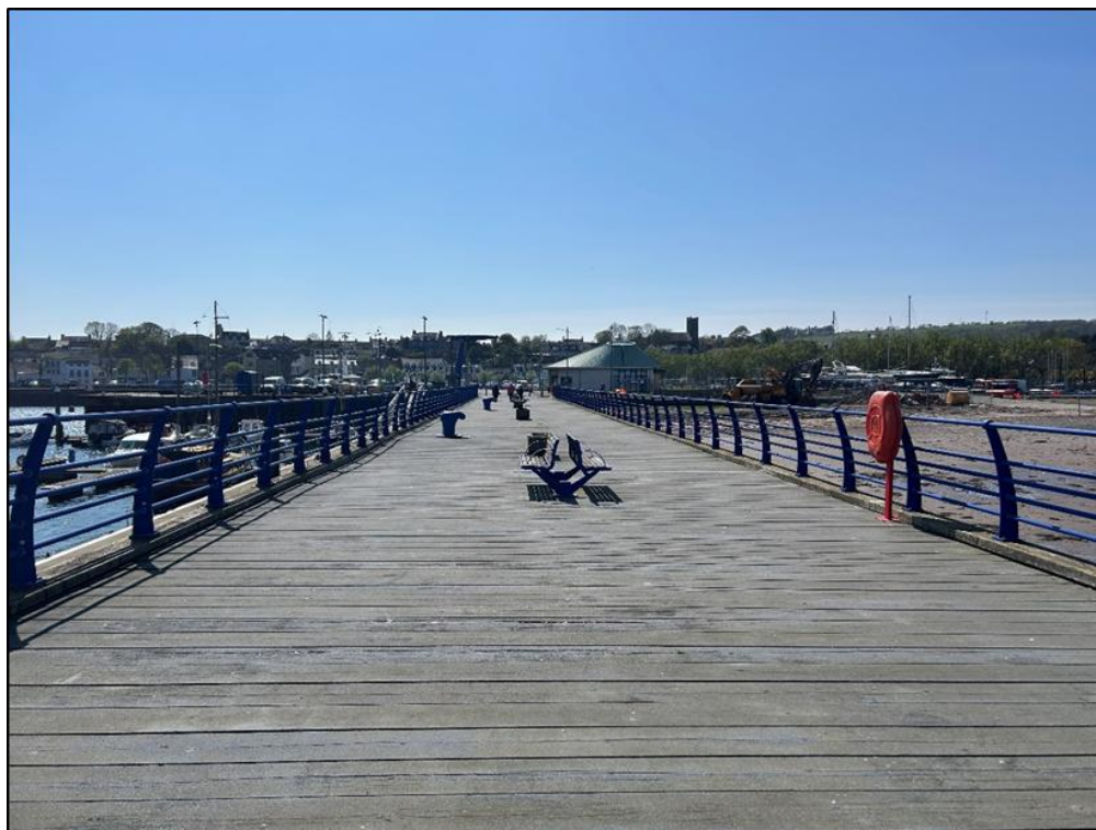
Photograph 8: View from West Pier back towards Harbourmaster building
