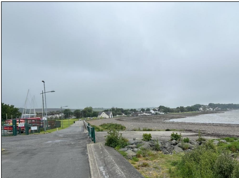
Photograph 1-4: View from Coastal Walkway path towards the beach and existing slip way to the west of the existing Marina
