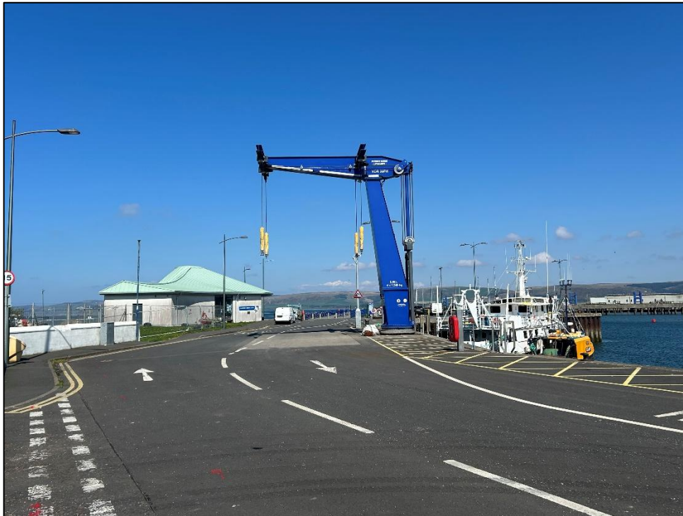
Photograph 1-3: views from access road towards existing Pillar Crane and Harbourmaster and Coastguard building
