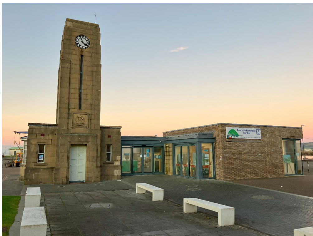
Photograph 22.1 Harbour Office with weighbridge (LB49655), viewed from the south
