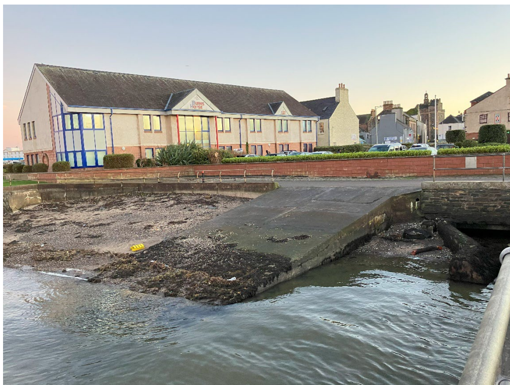
Photograph 22.1 Rear of 28 and 30 Harbour Street (LB41768) viewed from the north-west
