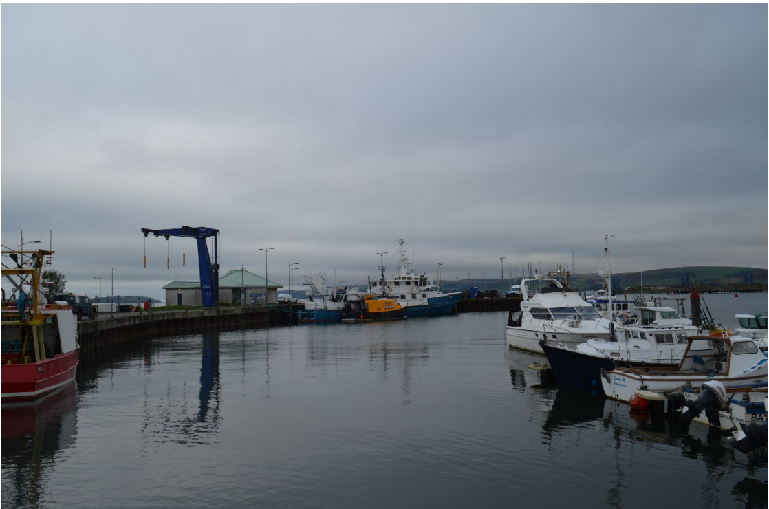
Photograph 23.5: View from the Coastal Path across the Marina to West Pier and the harbour office
