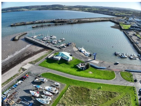
Photograph 3-1: Existing infrastructure in the harbour
