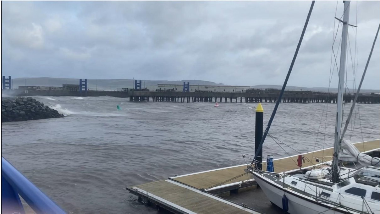
Figure 2.4 Storm waves entering Stranraer harbour 7 th December 2024.
