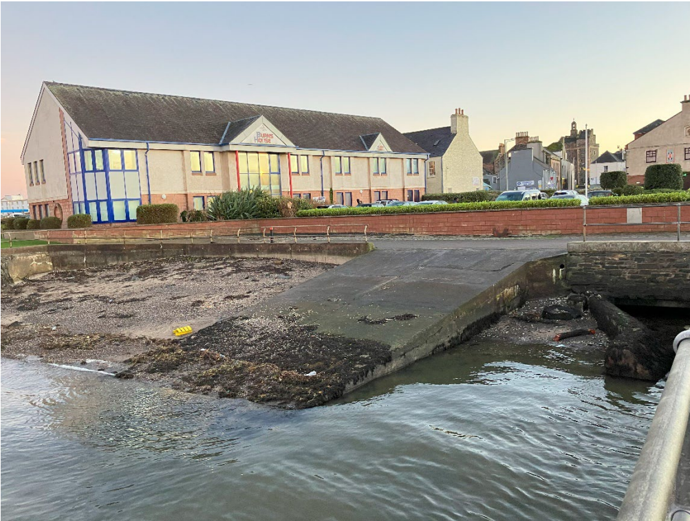
Plate 11 Rear of 28 and 30 Harbour Street (LB41768) viewed from the north-west
