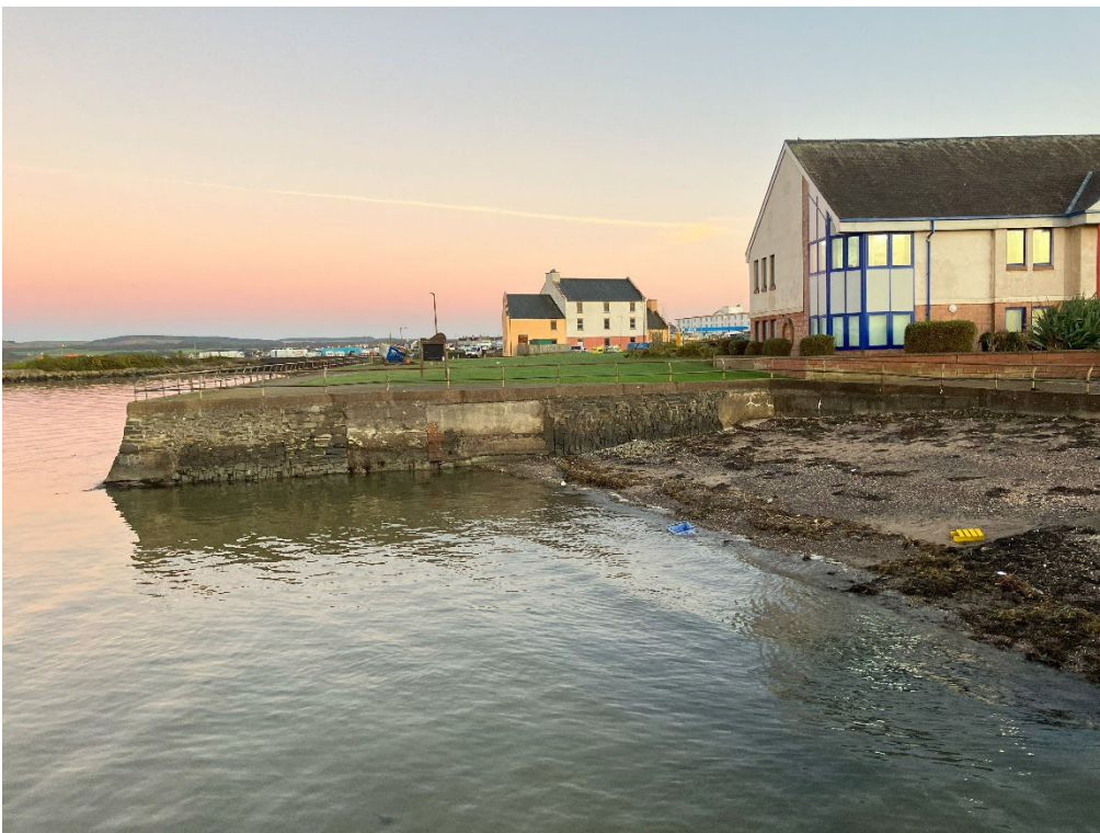
Plate 14 Harbour wall, looking east
