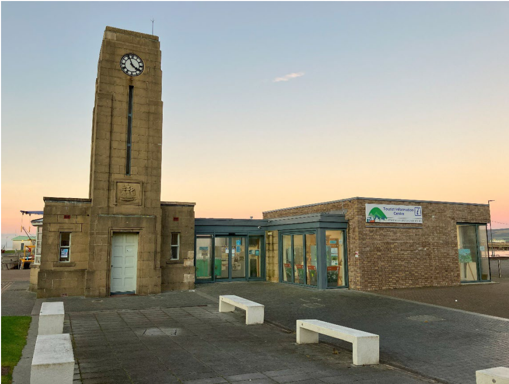
Plate 1 Harbour Office with weighbridge (LB49655), viewed from the south
