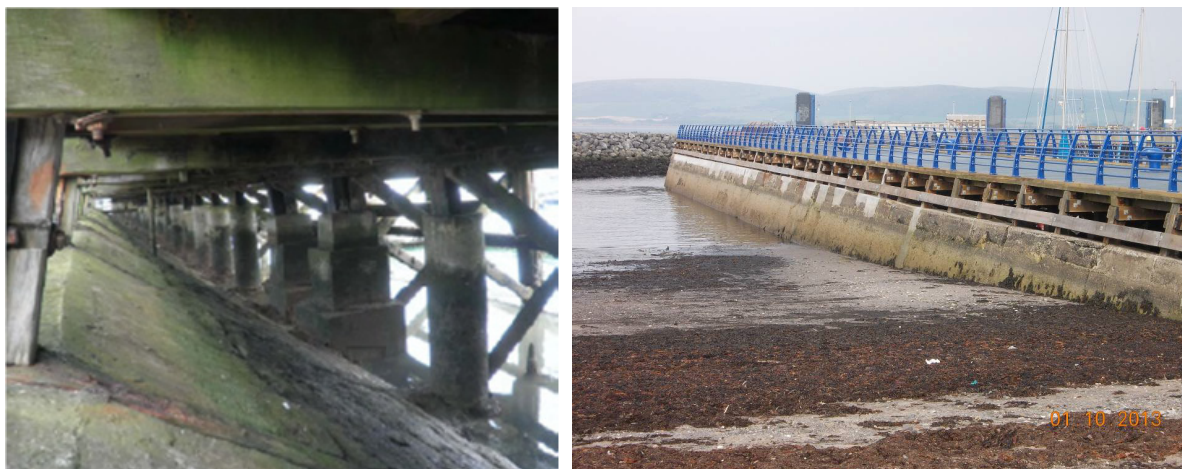
Figure 7-10: Photograph under and looking along the West Pier
