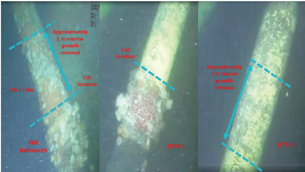
Figure 1-1 J-tube subsea survey images (F06 and OTM 1 ends)
