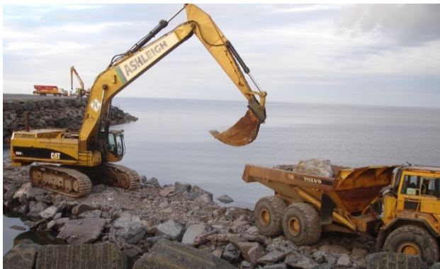
Plate 3: Excavator unloading from dump truck.
