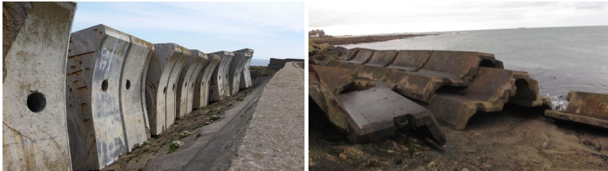
Figure 2-5 Photographs of large precast concrete units placed on the pitched revetment to encourage wave energy dissipation. (L) At the top of the revetment in front of the seawall. (R) At the bottom of the revetment before the toe.
