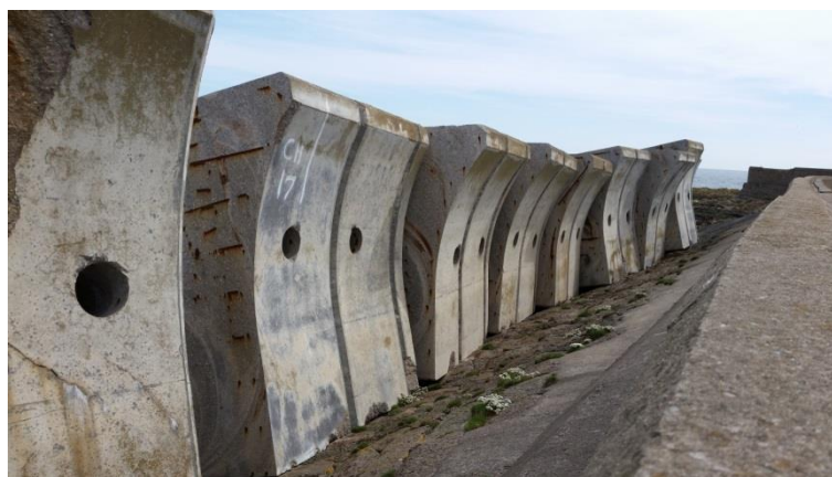
Figure 5-1 Large free standing concrete blocks along the pitched revetment (photo taken from the crest of the seawall looking easterly)
