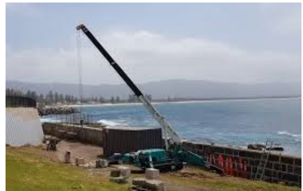
Plate 4: A crane for lifting units/armour into place or clearing existing revetment.
