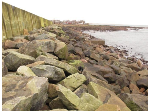
Figure 2-6 Photograph of the rock armour revetment taken from the end of the pitched revetment section
