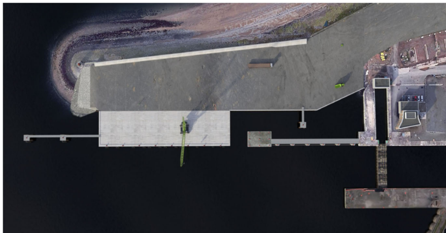
Finished Jetty development
