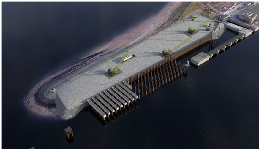
Placement of precast beams on the piles
