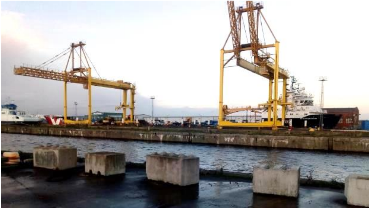
Figure 11-7 View across Imperial Dock Lock towards flight Sector 3, with gantry cranes and lighting columns in the background (photo courtesy of T. Edwards)
