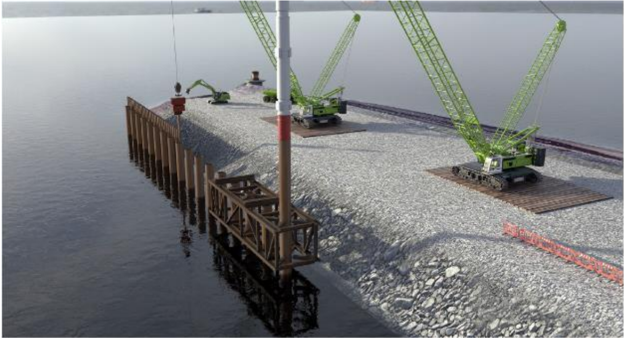
Figure 3-4 Installation of the piles
