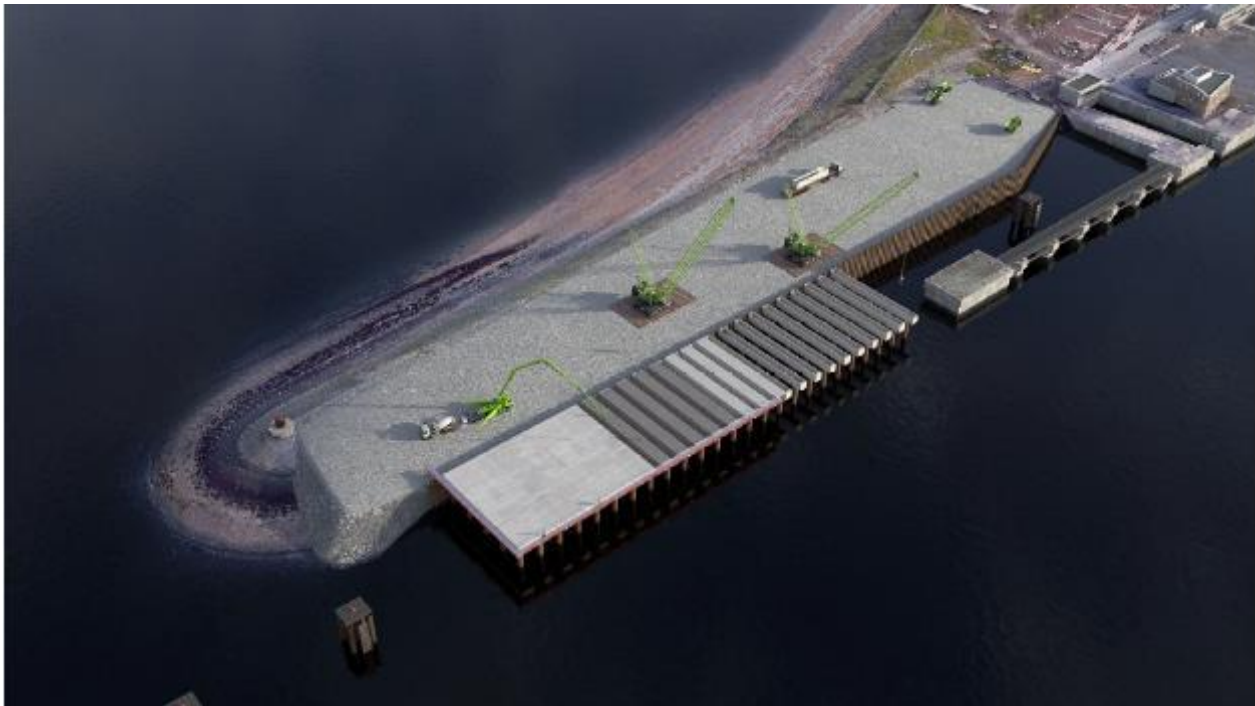
Figure 3-5 Placement of the precast beams, omni planks and pouring of the concrete deck
