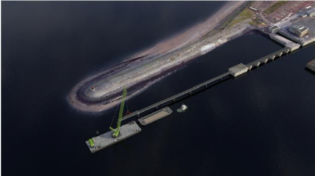
Figure 3-3 Removal of existing infrastructure
