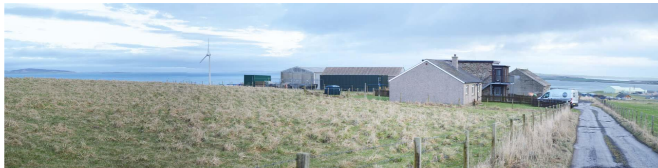
Figure 7.11 View from the northern edge of Hatston Park towards Hatston Farm and Hatston beyond
