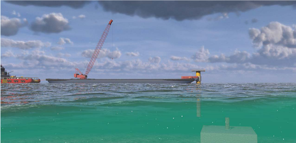
Figure 2-7. The barge has hold of the monopile and platform in the gripper with use of chain pullers
