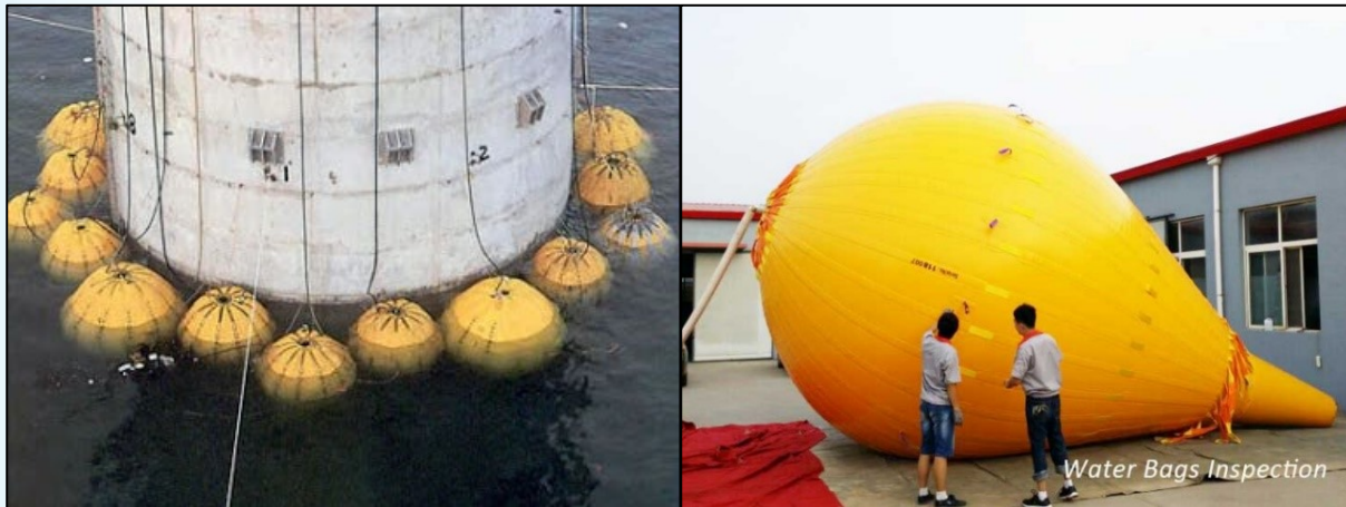
Figure 2-10. Example of airbags being used to re-float an underwater structure.
