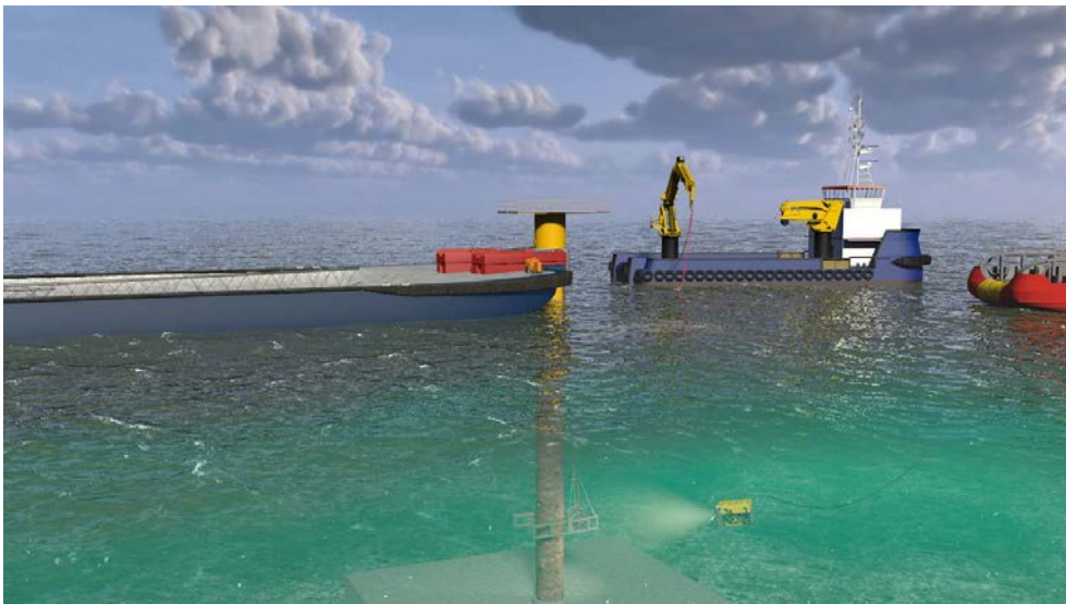
Figure 2-6. Cutting supported by WROV from support vessel
