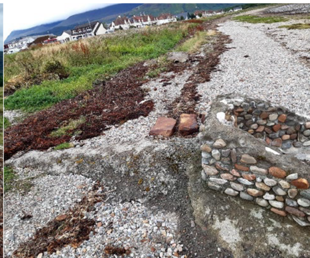
Figure 2.6: Landward End Of The Existing Caol No1 Outfall
