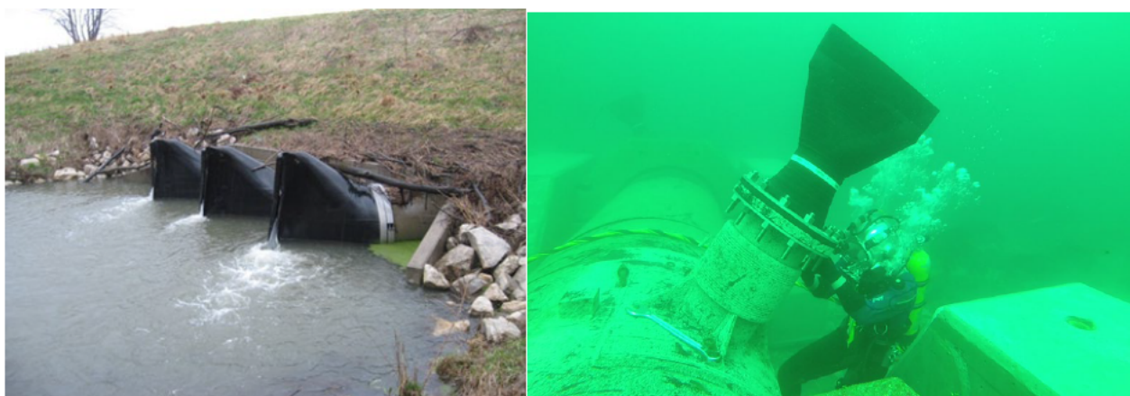
Figure 3.1: Examples of a duckbill non-return valve
