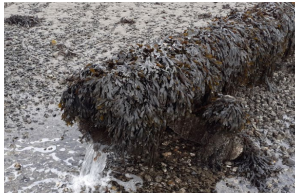
Figure 2.4: Existing Caol Transfer Outfall Discharge End
