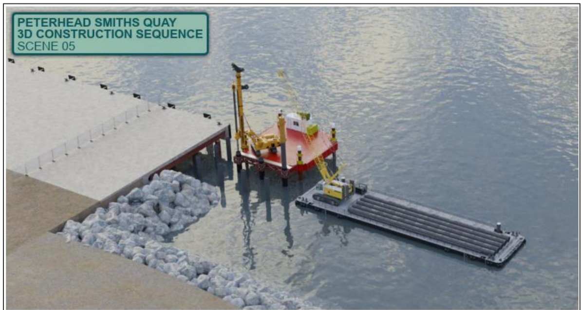
Figure 2.5 Pile installation from jack-up barge.
