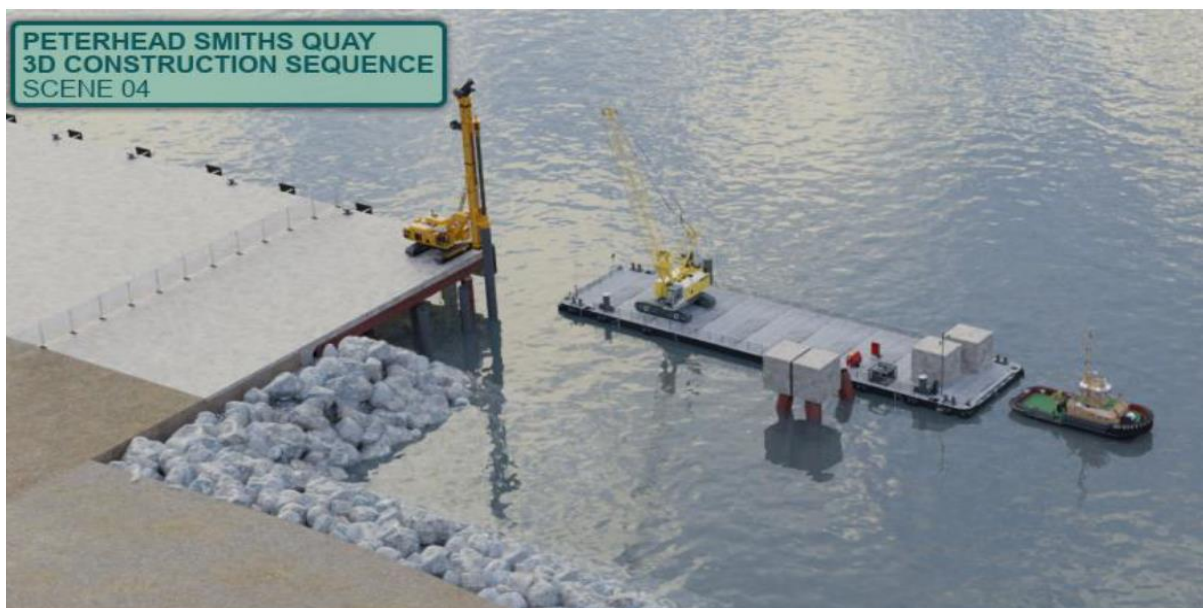
Figure 2.4 Initial pile install working from Smith Quay.
