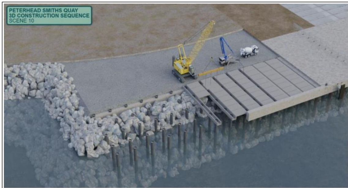
Figure 2.8 Placement of trough beams and precast deck planks.
