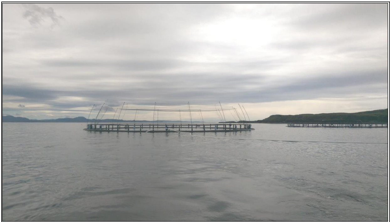
Figure 7: PROPOSED: Photo of a circular pen with poles at the walkway to support the top/bird netting.
