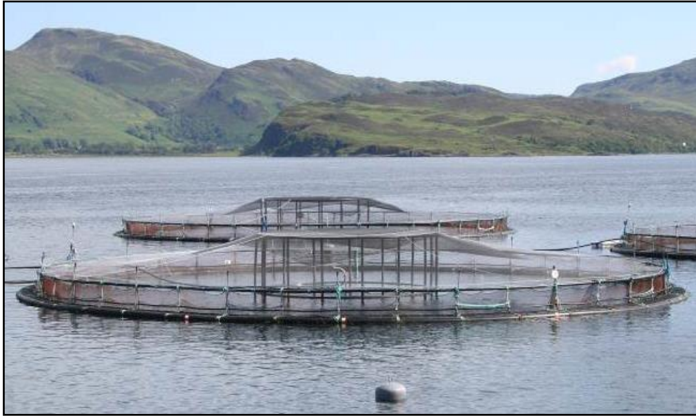
Figure 6: EXISTING: A photo of a circular pen with a hamster wheel, showing the Sinker Tube technology which improves net tensioning and pen structure. The inner surface plastic ring is a float which holds the bird net above the water surface. The lower plastic ring is the weighted sinker tube, with chains rising to the surface plastic collar.
