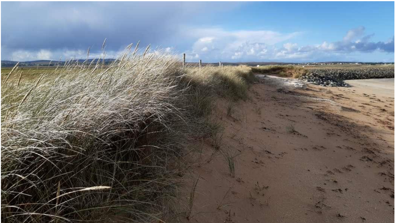
North-western end of beach – transition from beach to rock armour
