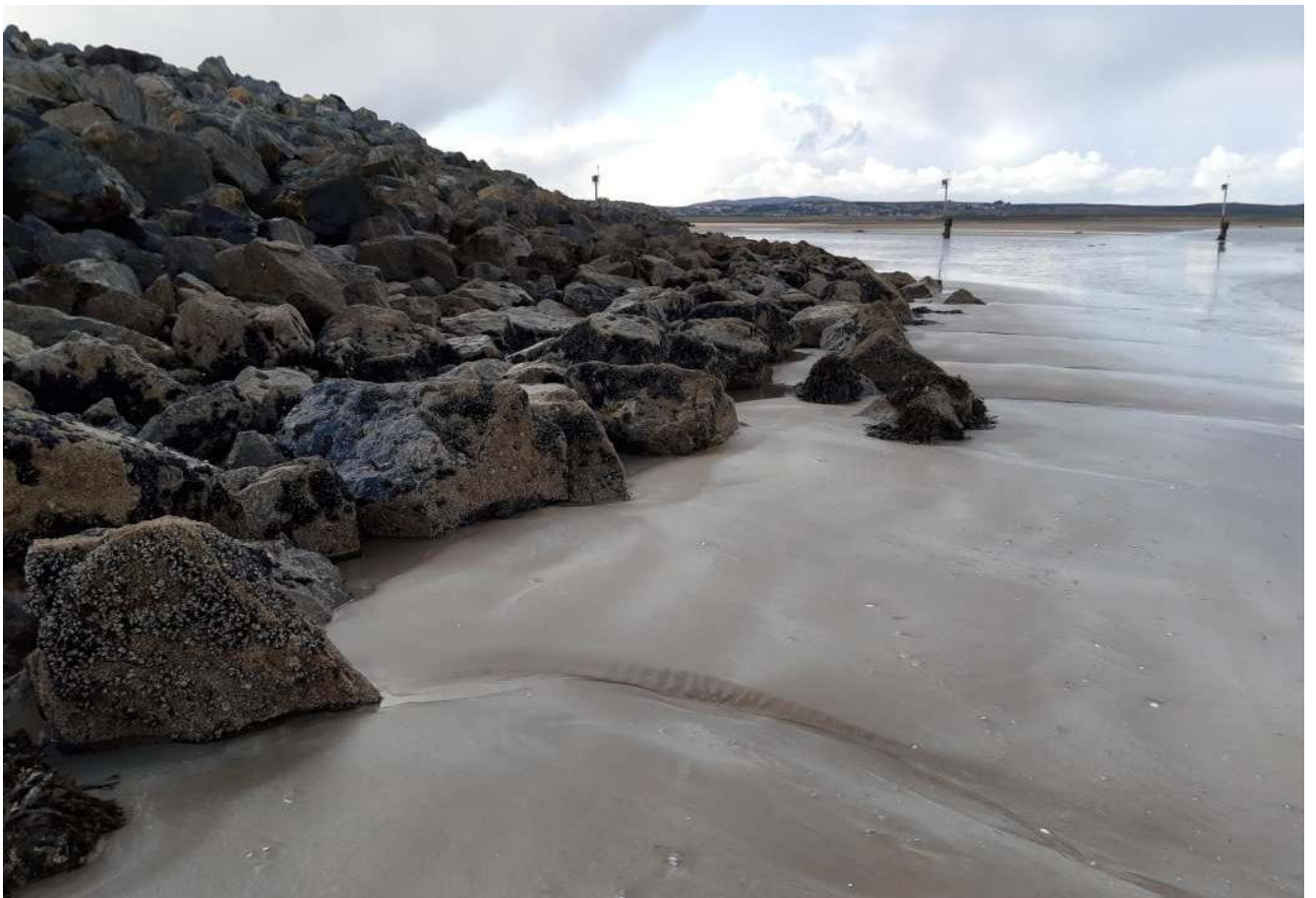
Northern end of rock armour headland
