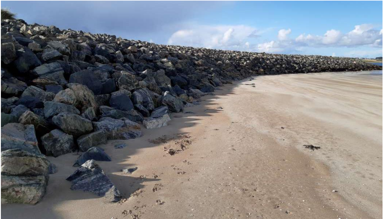
Eastern flank of Rock Armour Headland
