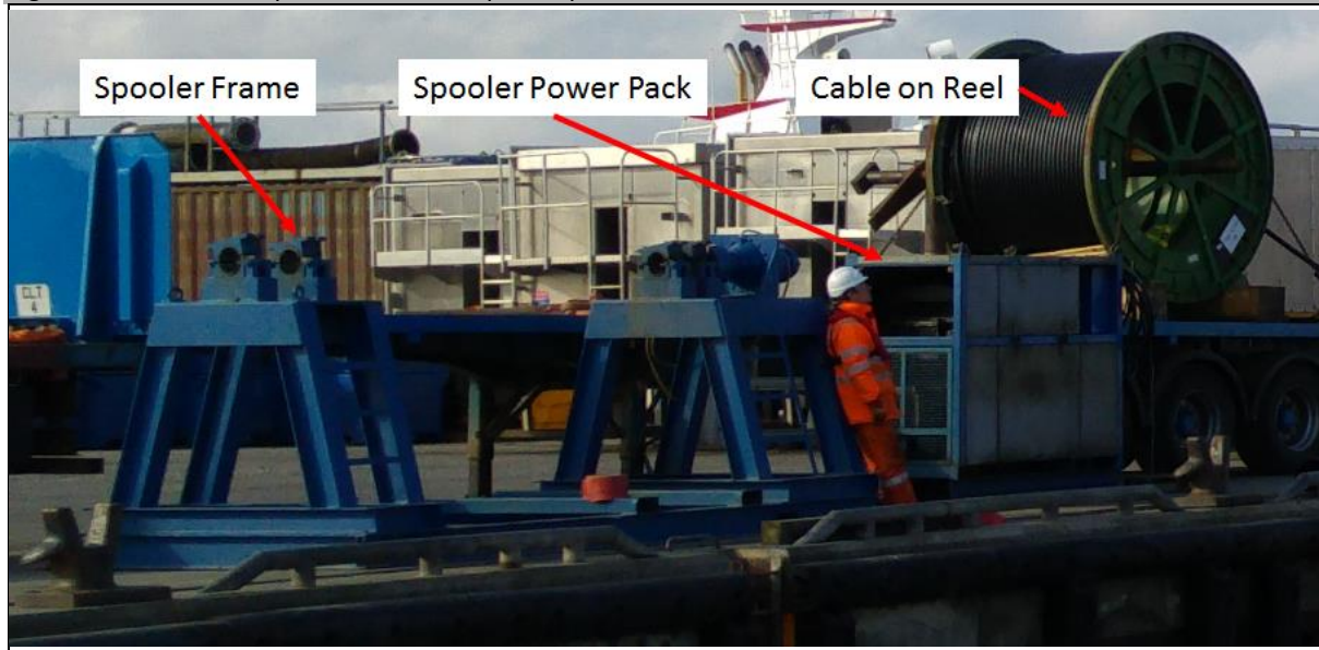
Figure 4.2 Cable reel, spooler frame and power pack
