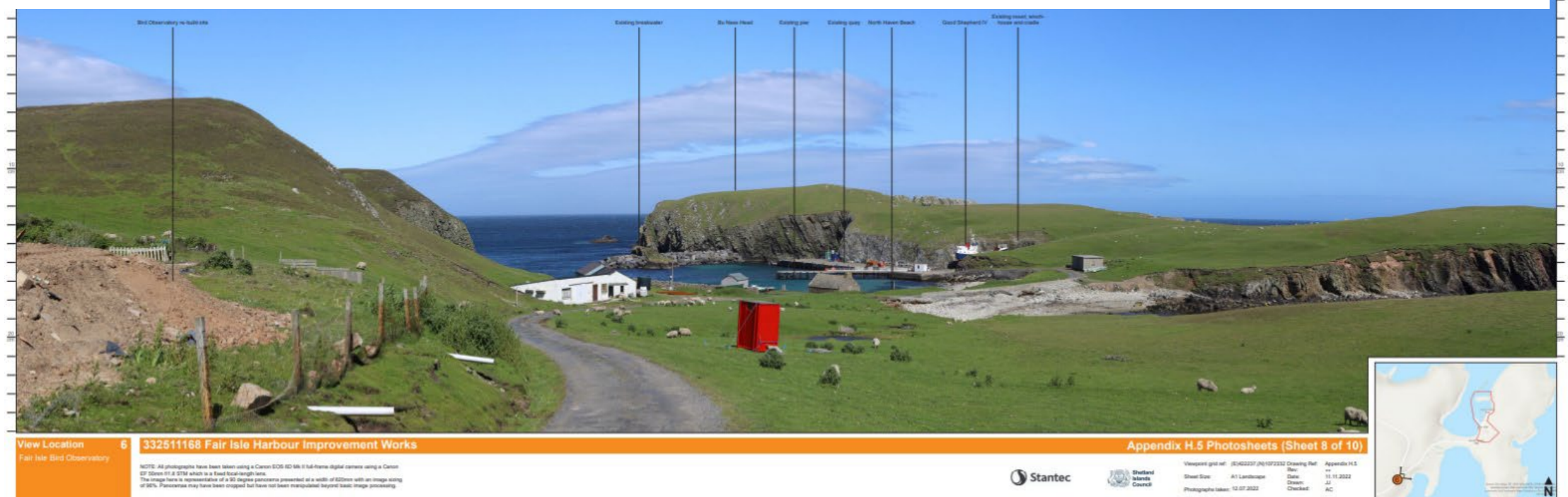
Figure 7 - View of Fair Isle Harbour Facing North from the Access Road
