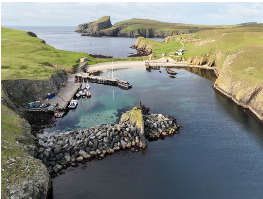
Figure 3-2 North Haven harbour
