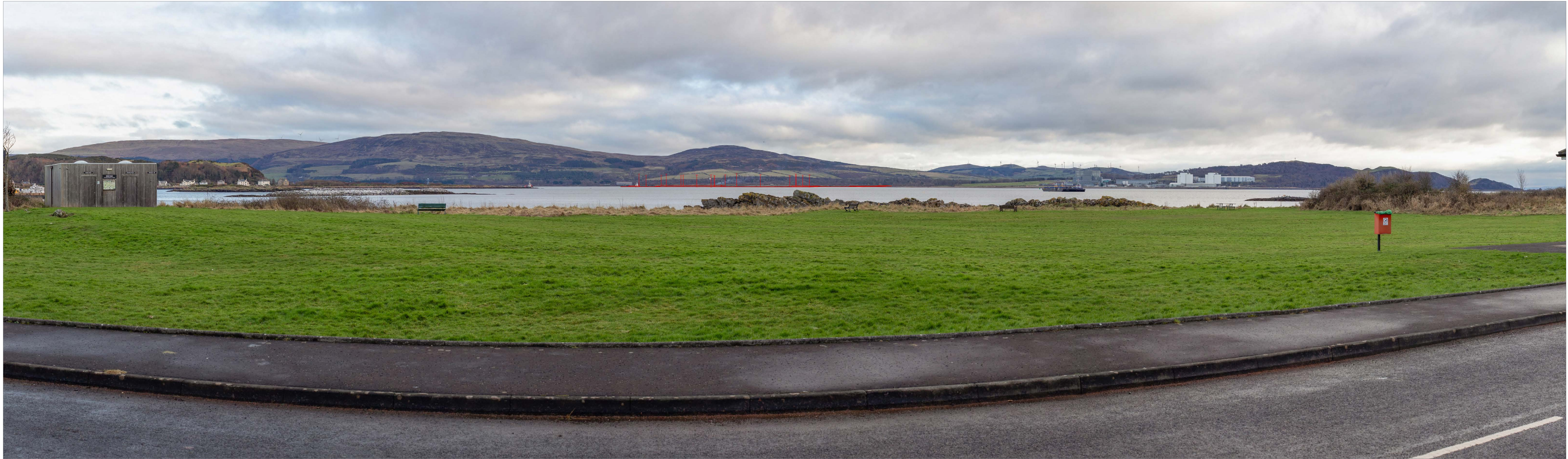
Hunterston Construction Yard - EIA - Viewpoints Figure 6.6.9b - Viewpoint 9: W Bay Road, Millport Viewpoint
