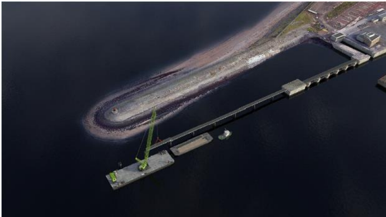
Figure 2-3 Removal of existing infrastructure
