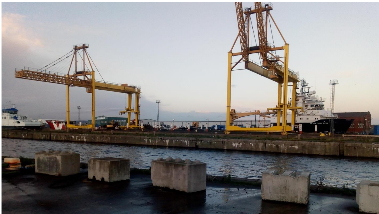
Plate 7.1 View across Imperial Dock Lock towards flight sector 3 (Jennings, 2012), with gantry cranes and lighting columns in the background (photo courtesy of T. Edwards)
