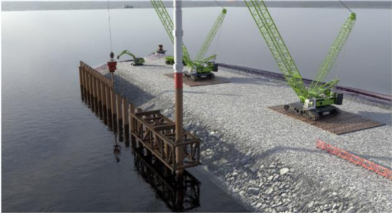
Figure 2-4 Installation of the piles
