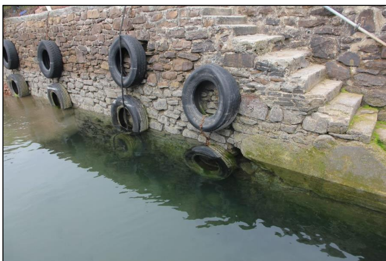
Image 3 Southeastern view of the pier
