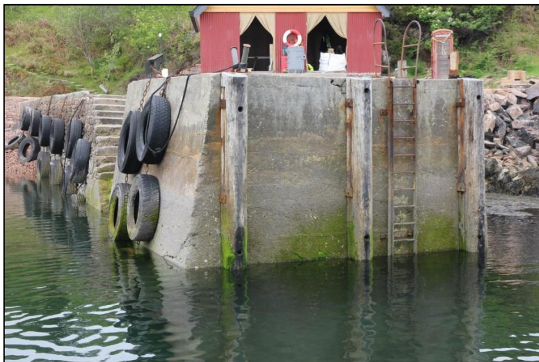
Image 2 Northeastern view of the pier
