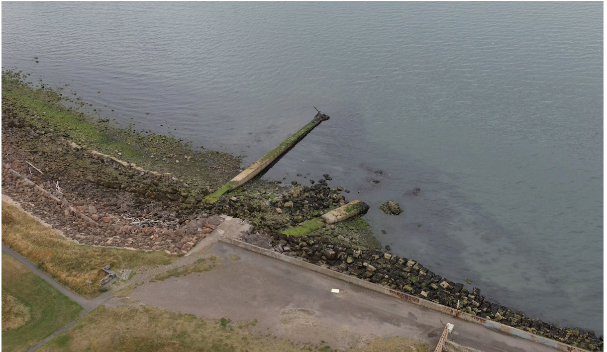
Figure 7.1.2 Detail of the seawall and rock revetment
