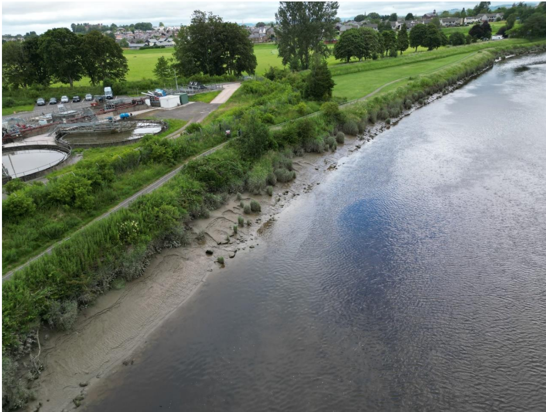
Photo 4 (below): Failing embankment adjacent to southern (downstream) end of WwTW
