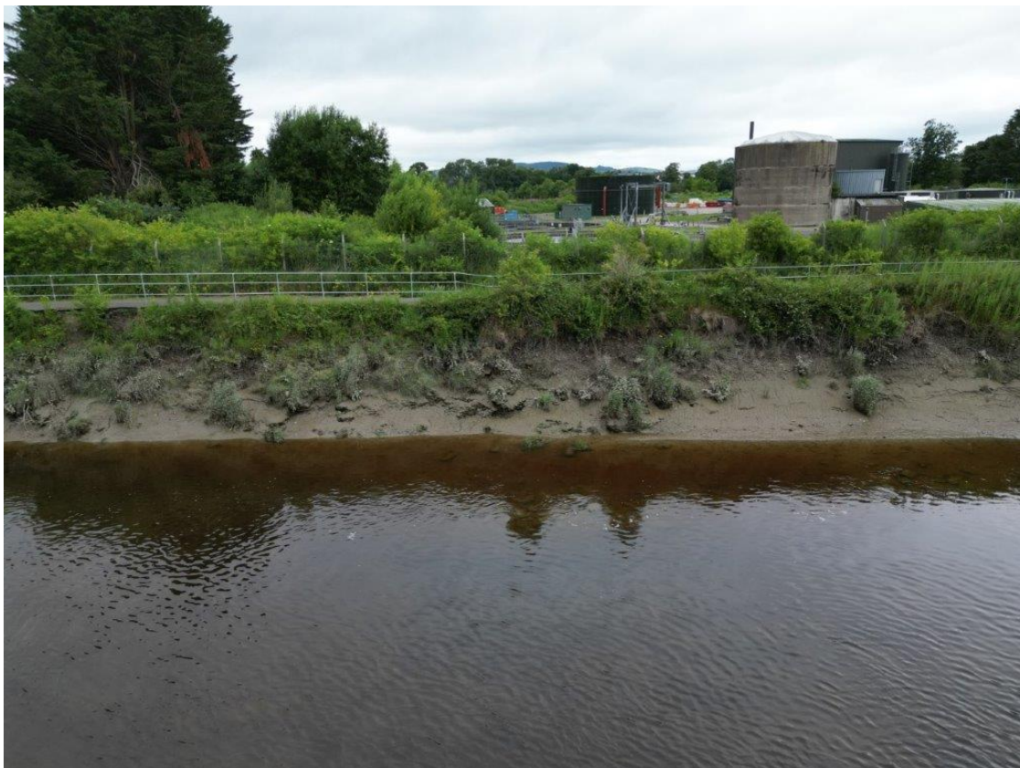
Photo 4 (below): Failing embankment adjacent to southern (downstream) end of WwTW
