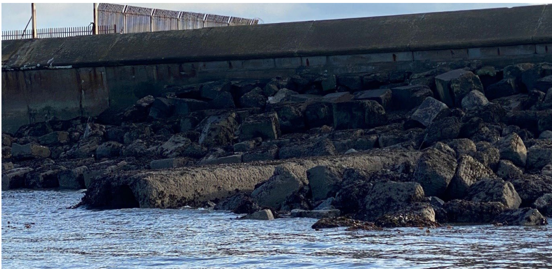
Figure 2.1: Existing ELC Outfall
