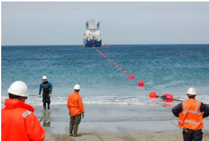
Figure 2-11 Typical DSE landing from MLV
