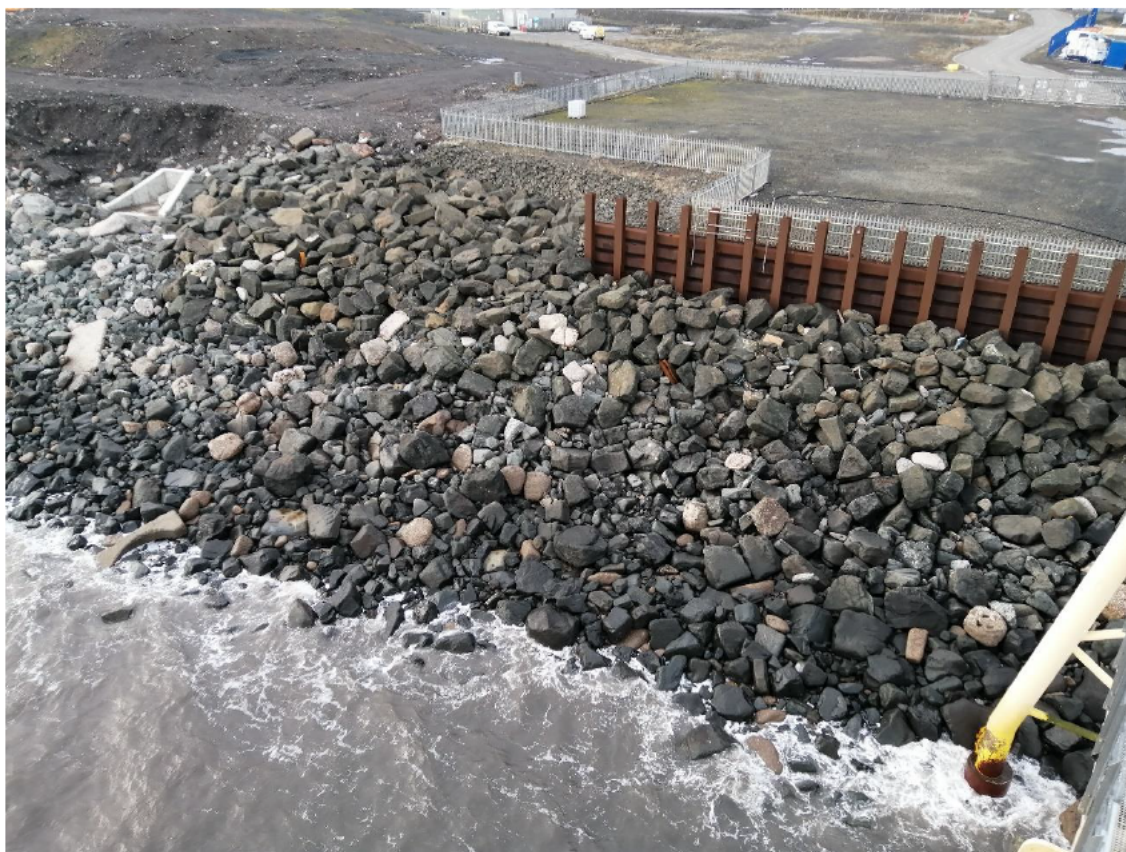
Figure 1: Western section of revetment reconstructed in 2016 (taken: 22/11/2023)
