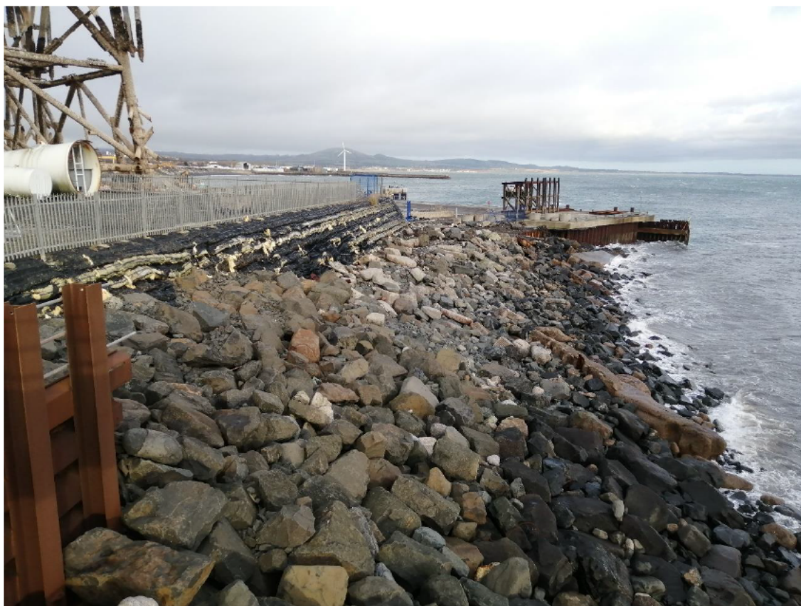
Figure 6: Eastern section of revetment reconstructed in 2016 (taken: 22/11/2023)
