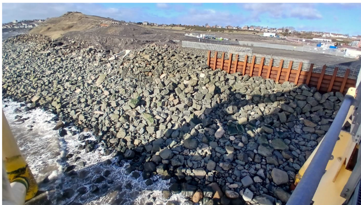
Figure 2: Western section of revetment reconstructed in 2016 (taken: 29/02/2024)
