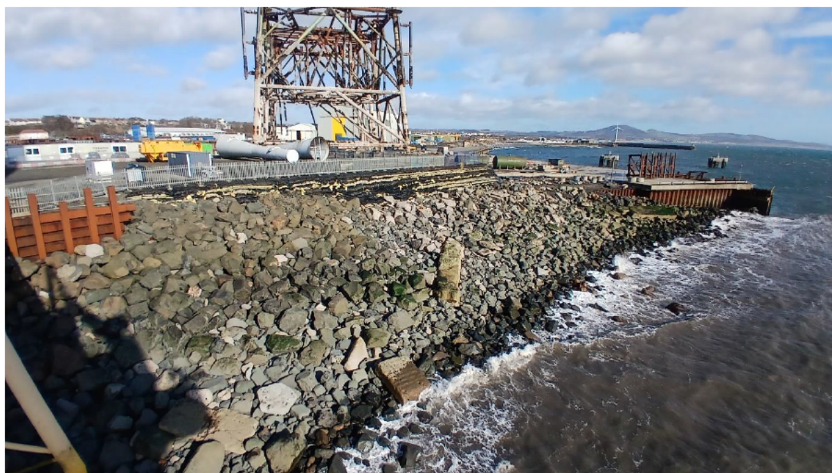
Figure 4: Eastern section of revetment reconstructed in 2016 (taken: 29/02/2024)
