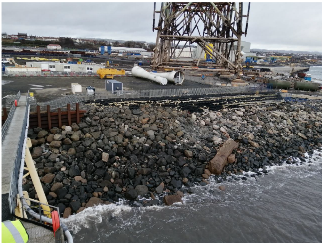
Figure 3: Eastern section of revetment reconstructed in 2016 (taken: 22/11/2023)
