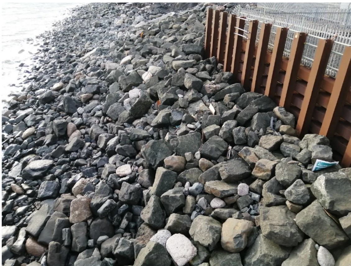
Figure 5: Western section of revetment reconstructed in 2016 (taken: 22/11/2023)
