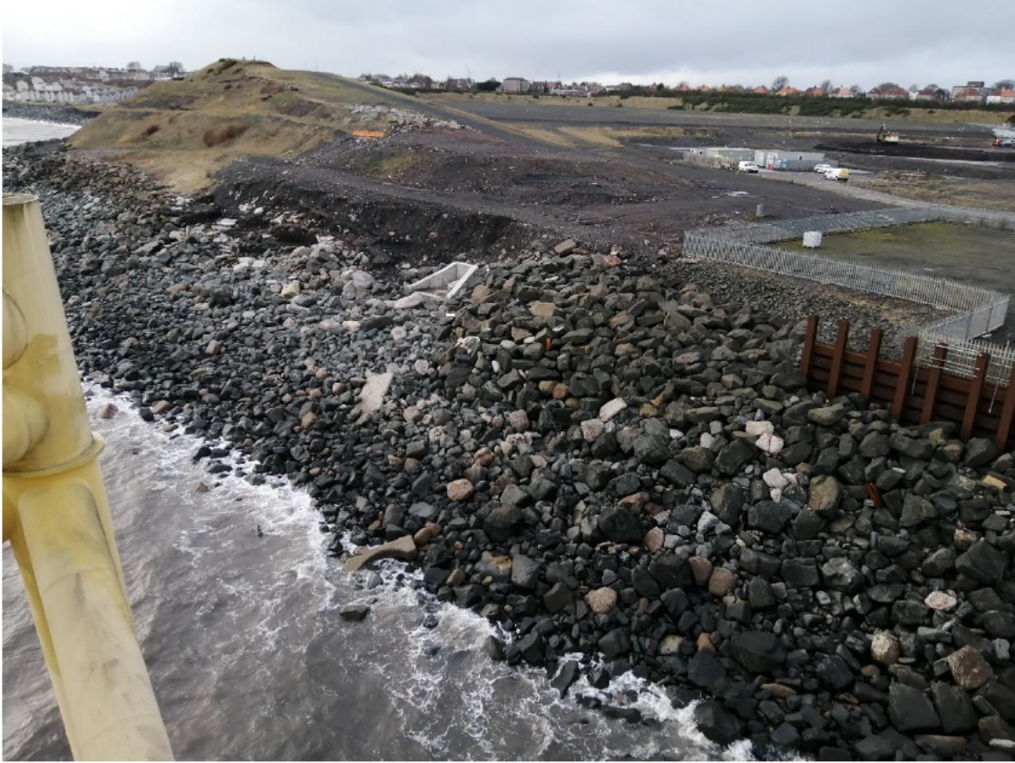
Figure 7: Western section of existing revetment (taken: 22/11/2023)
