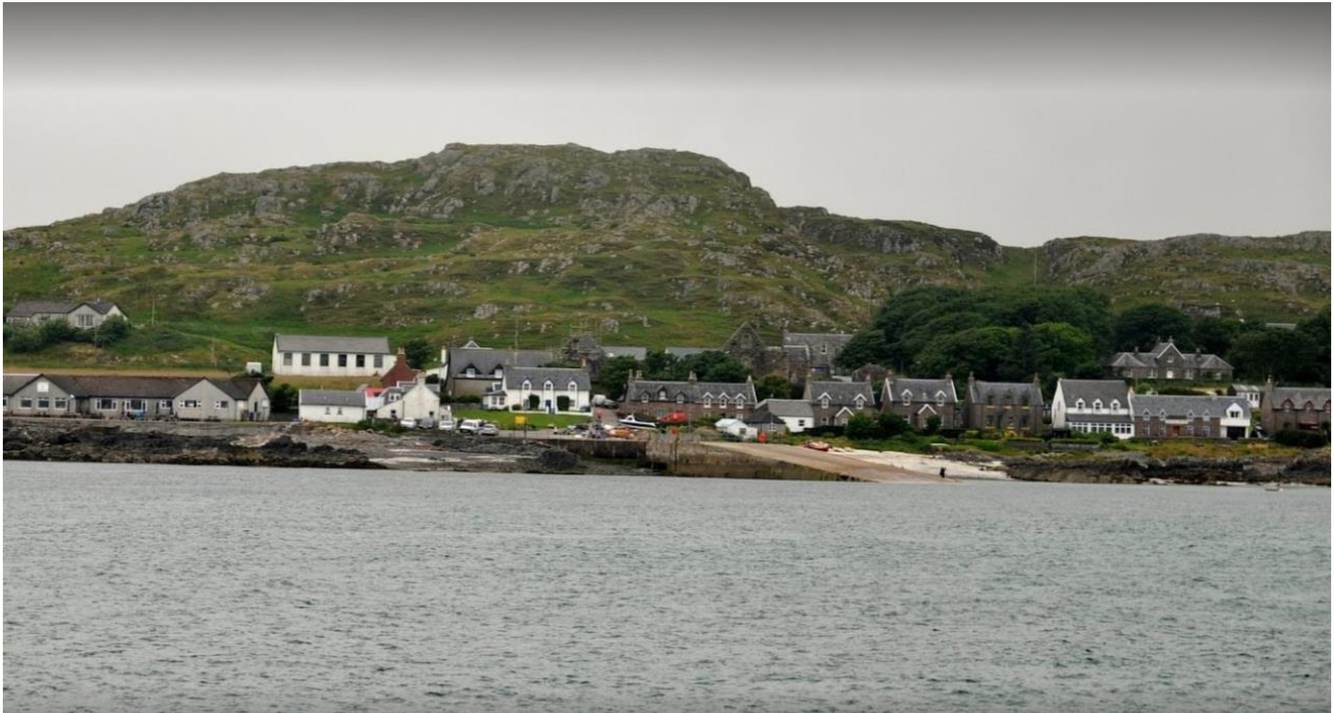
Figure 3-2 Iona slipway ( Image Source: Google.com (dated July 2018) )
