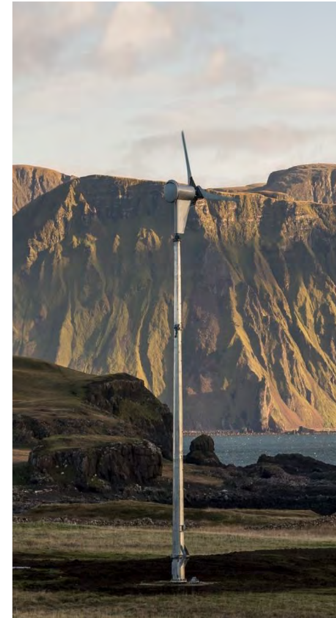
12-15kV turbine. Approx. 15m high.
