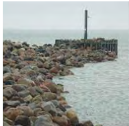
Example image of rubble breakwater
