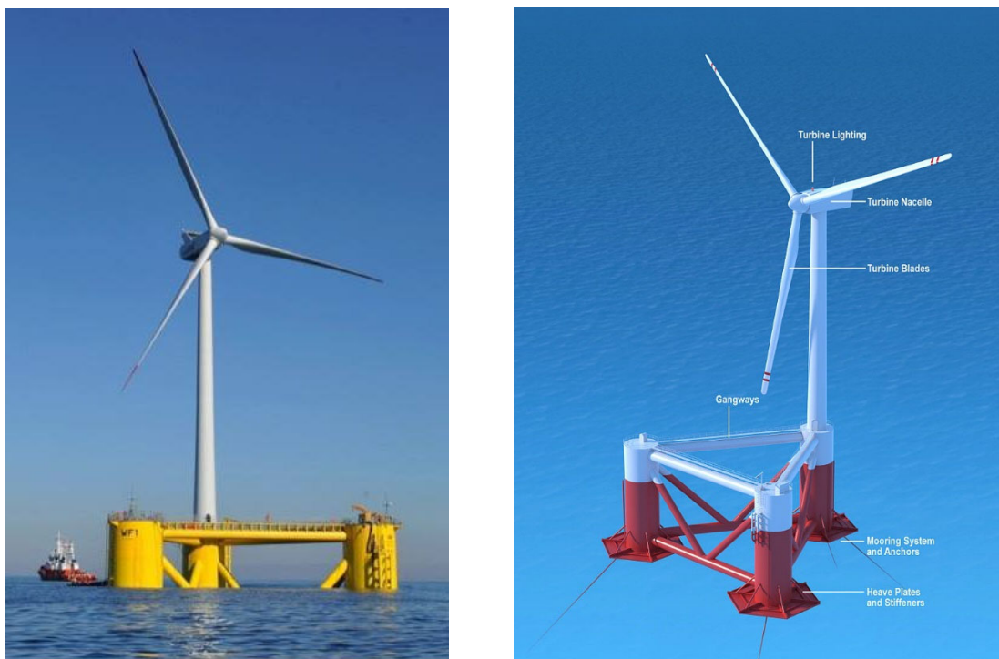
Figure 4-5 Windfloat™ Steel Semi-Submersible
