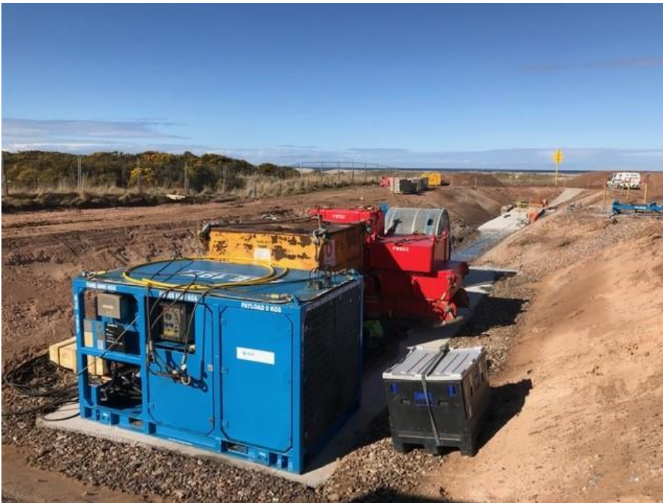
Figure 2.8 - Cable Pull-In Winch
