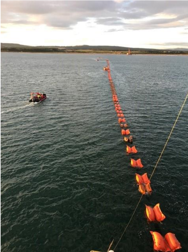
Figure 2.6 - Cable Float In
