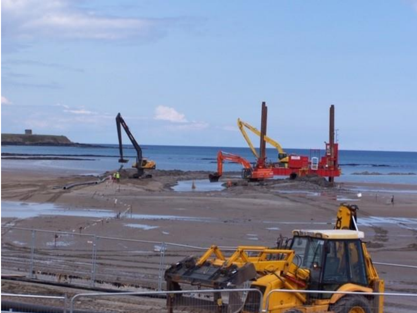
Figure 2.5 - Open Cut Trenching
