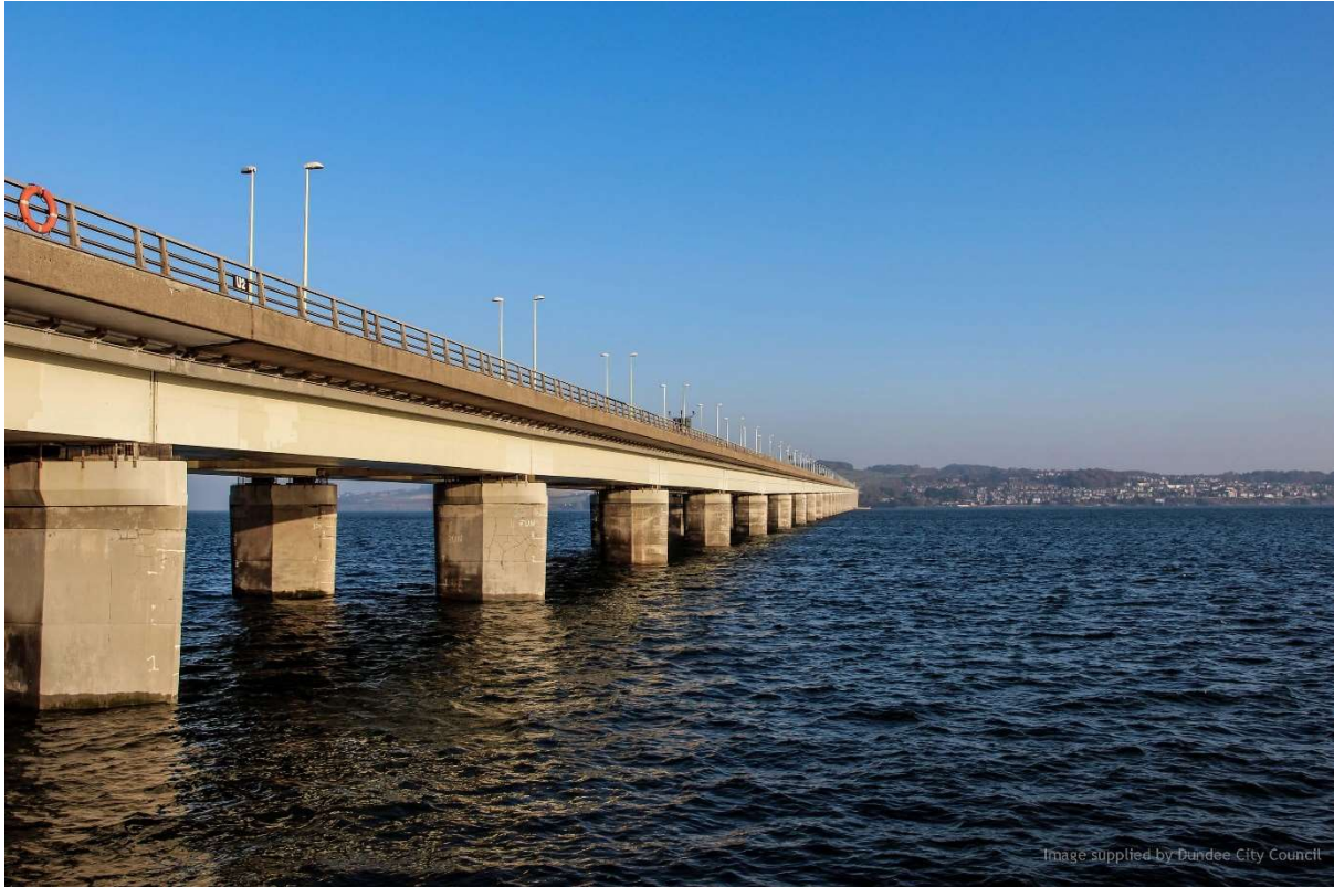
General View of Tay Road Bridge from Dundee Quayside (looking Southeast)
