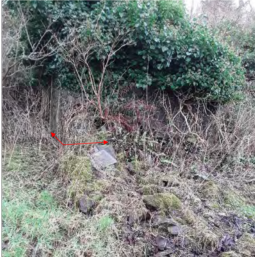
Photograph 3 – Onsite overground ruined historical residential property close to western boundary (red arrows represent a corner of the property)
