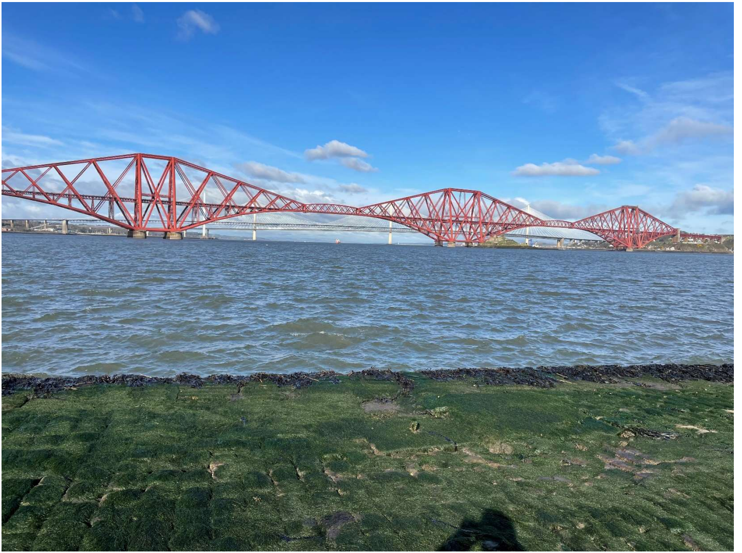
4. The Three Bridges to the West of Longcraig Pier
