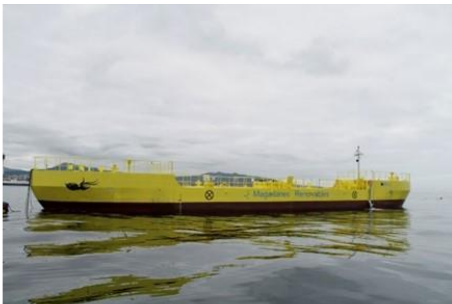
Figure 6: External View of the Platform (Upper Block)
