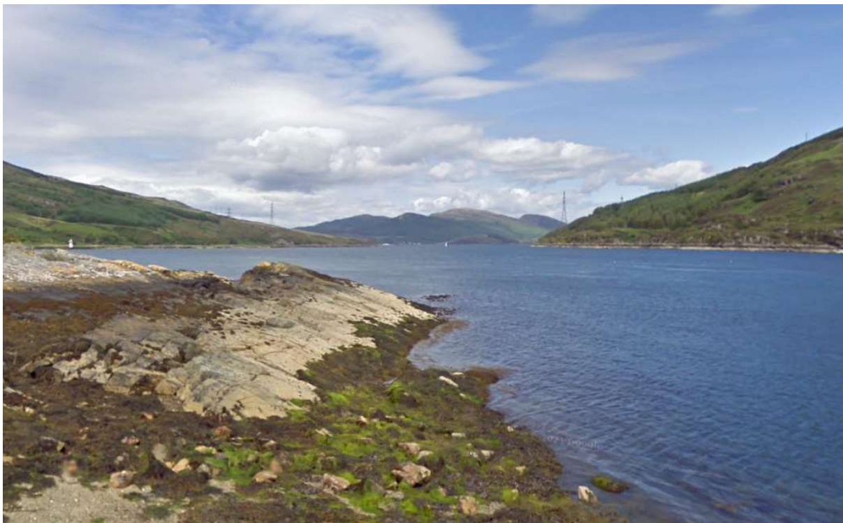
Figure 4-1: View of the overhead line spanning Kyle Rhea, from the ferry crossing
