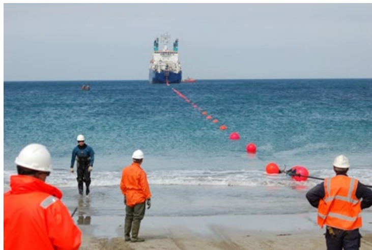
Figure 2-16 Typical direct shore landing from MLV
