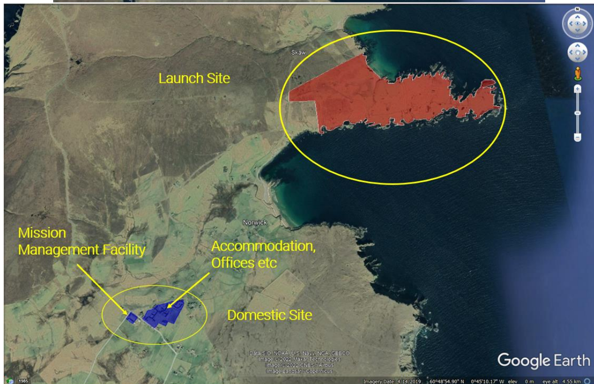
Figure 1 Lamba Ness Launch Site and Mission Management Facility in relation to each other.
