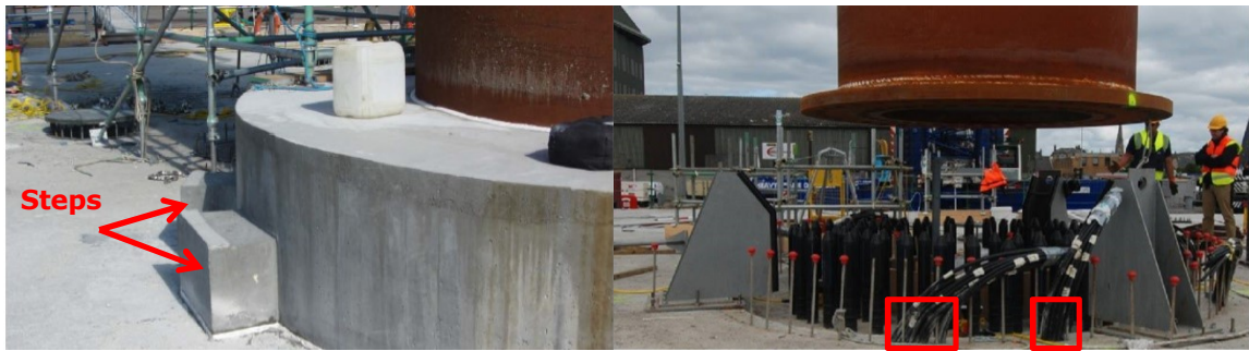
Figure 3. Steps casted to plinth
