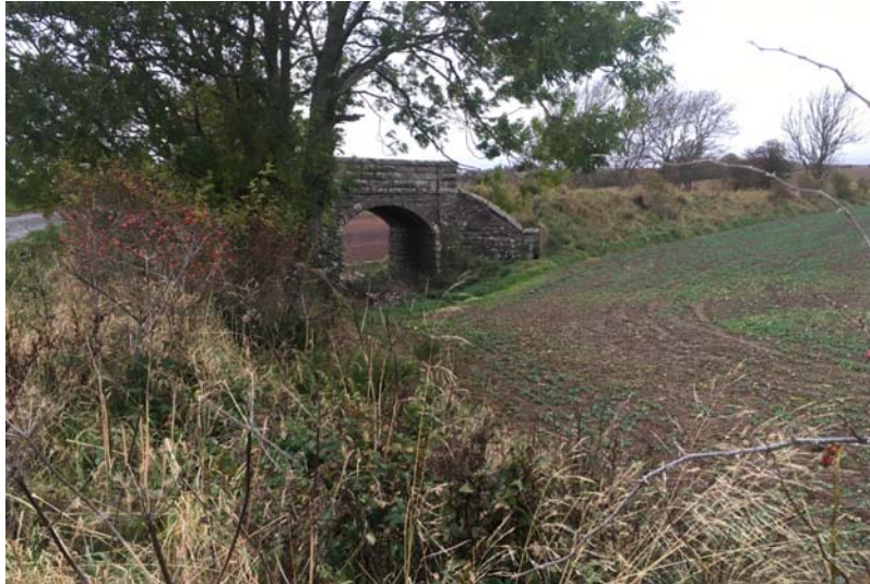
Figure 9 - Existing Bridge on Access Road
