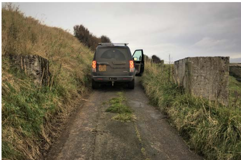
Figure 10 - Existing Tank Stops on Access Road
