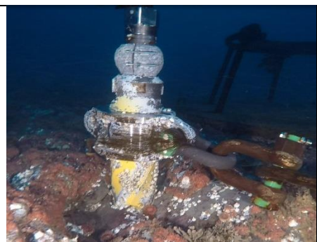
Fig 5 c) Shackle Type connection on anchors 2,3,4
