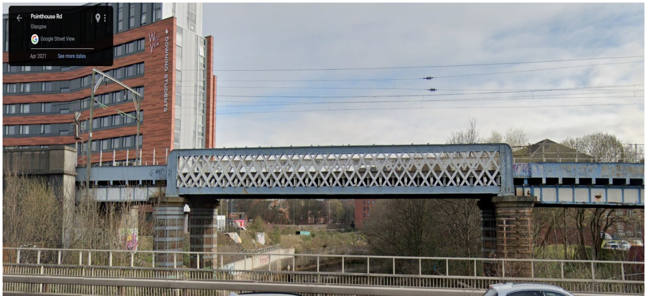
Figure 1 – UB240/131 Kelvin Viaduct (Street View o- north facing)
