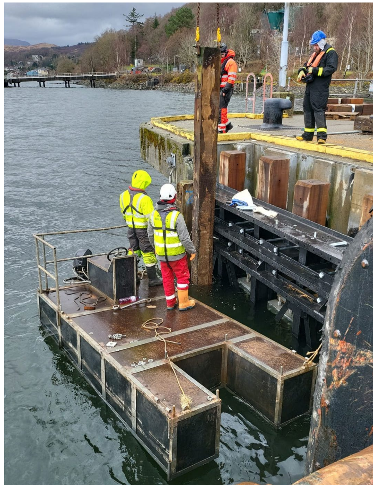
Figure 3 – Garelochhead Fender Strong Backs Refurbishment
