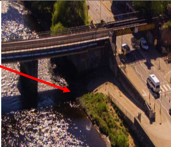
Figure 1. Slipway at Tay Viaduct on West Side
